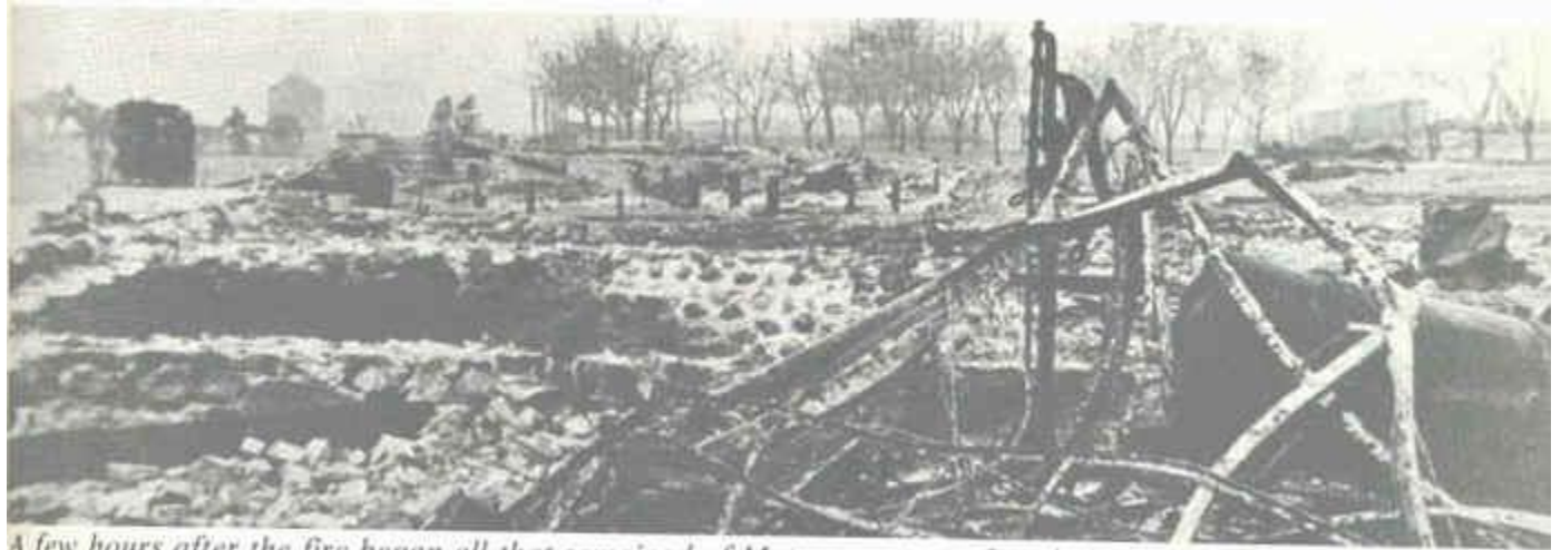
A few hours after the fire began all that remained of Metz were stone foundations and twisted metal.
